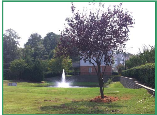
Photo of the retention pond stormwater device at Brook Forest in Raleigh. Storm water is routed from storm drains on the property to the wet pond where it stores the runoff, settles out sediment, removes parking lot oil, grease and excess fertilizer.
